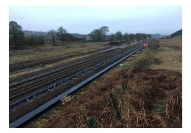
New troughing route alongside railway required for signalling equipment. The troughing also provides a safe walking route for railway maintenance teams .
