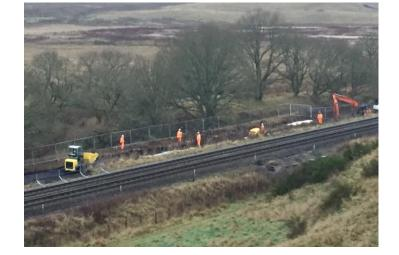
Haul route built alongside the railway will allow us to move equipment and materials to allow the construction of new railway embankment.
