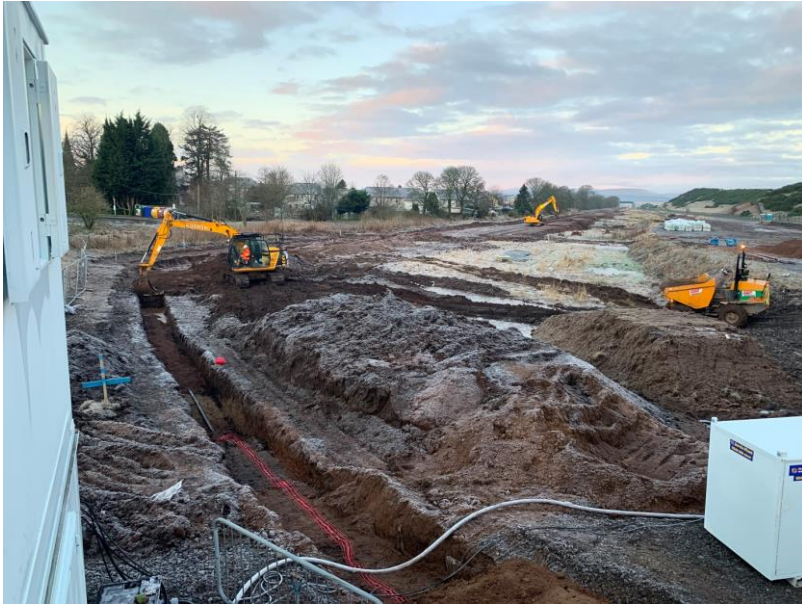
Backfilling Rising Main
