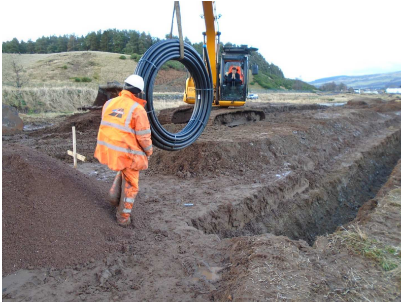
Installation of new Rising Main
