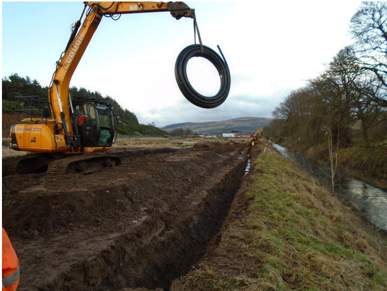
Installation of new Rising Main
