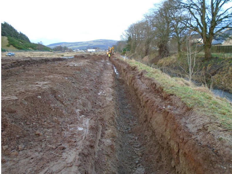
Excavation for new Rising Main
